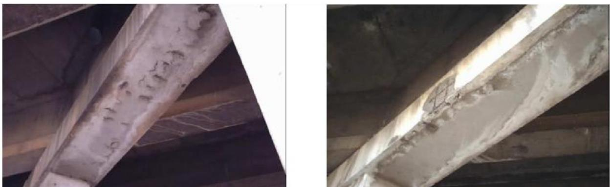
*Figure.I. 5: Insuffisance d'enrobage*
