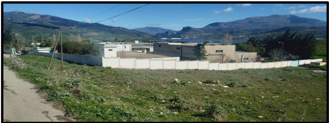
Figure (18) : Station d'épuration de sidi merouane.
