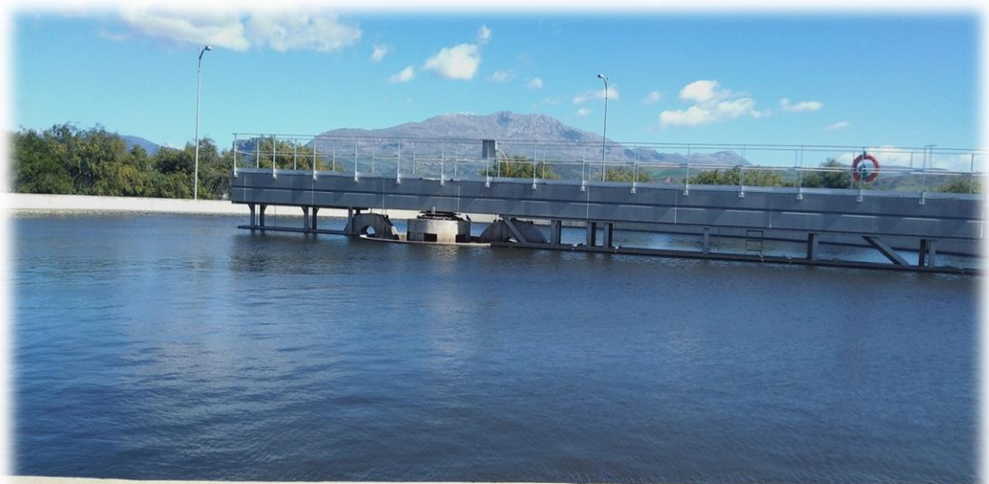
Figure (32) : Clarificateur.
