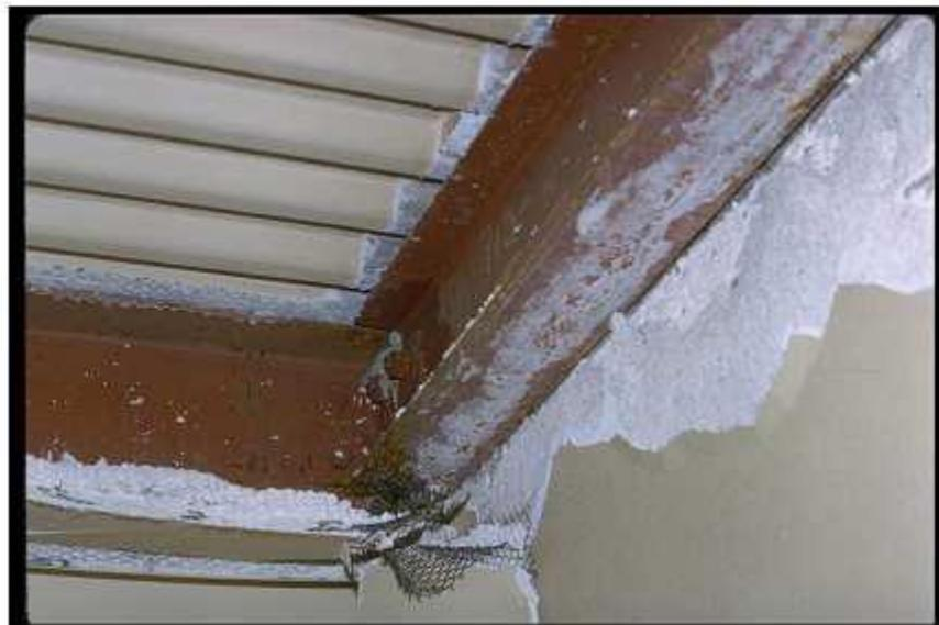
**Figure I.32.** Plancher collaborant.
